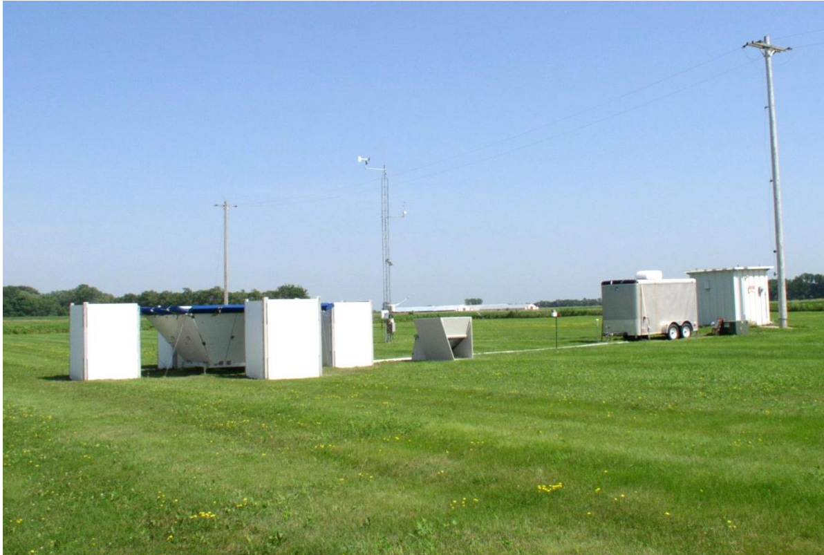
Figure 2.1. The WFIP 915 MHz wind profiling radar at Saint James, MN. The center enclosure contains the transmitter, a phased-array antennae, and a clutter-suppression screen. The four white rectangular boxes are the Radio Acoustic Sounding System (RASS) loud-speakers. The gray enclosure to the right of the wind profiler is a co-located sodar system, and a 10m mast with surface met instrumentation is visible between the profiler and sodar. The portable trailer contains the computer data acquisition system and communication equipment.
