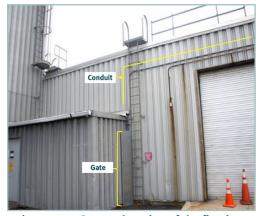
Two or more decades ago, a lockable sidehinged gate was installed to cover the bottom eight rungs of the ladder. The gate was intended to prevent access to the Lab 17 roof because of radiological exposure concerns during sample loading or removal in the building below. That exposure concern no longer exists, but the gate remains. In
