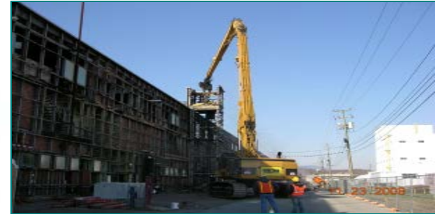
Elevator shaft being demolished
