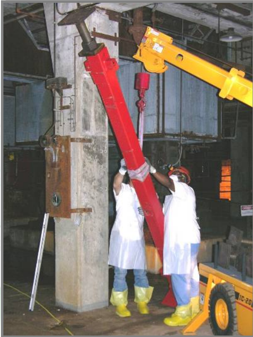
Crews installing a corbel repair
