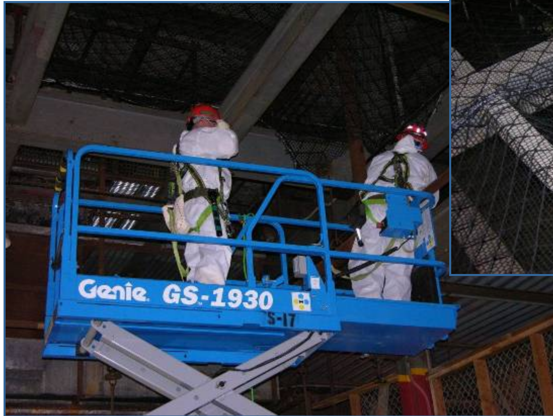
Crews installing protective nets and barriers
