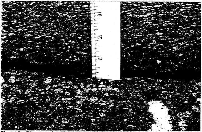
Figure 5 – Photograph taken March 11, 2004 showing area of heaved pavement highlighting area of vertical displacement > 1/4-inch.
