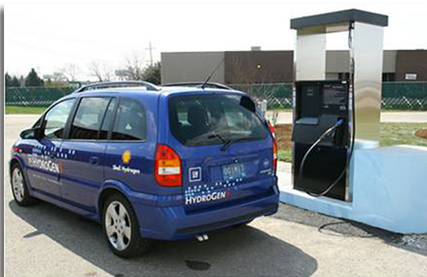
H2 ProGen Hydrogen Dispensing Station
