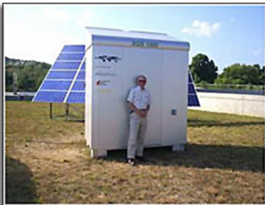
The Avalence Electrolysis Unit with Photovoltaic Array
