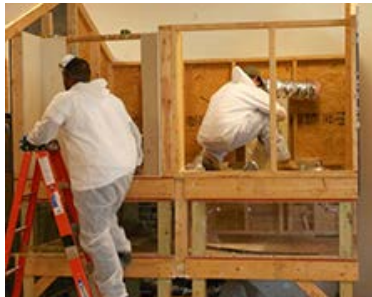
Trainees practice techniques on miniature model homes at the New River Center for Energy Research and Training in Christiansburg, Virginia.
