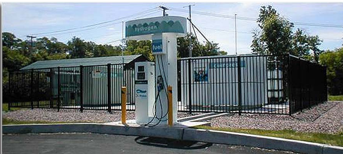
EVermont Demonstration Fuel Station in Burlington, VT
