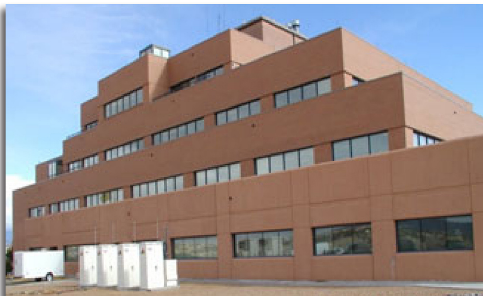
Plug Power's 5-kW GenCore Fuel Cell Provides Emergency Backup Power at the New Mexico National Guard Facility in Santa Fe
