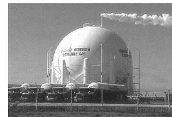
bigger is better. This heat causes some of the hydrogen to vaporize and the tank pressure to increase. Stationary liquid hydrogen storage tanks are often spherical since this shape offers the smallest surface area for a given volume, and therefore presents the smallest heat transfer area.
