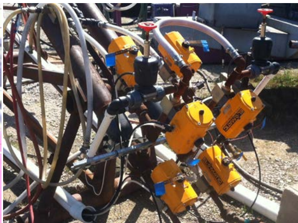
Pump Slurry Discharge Section
