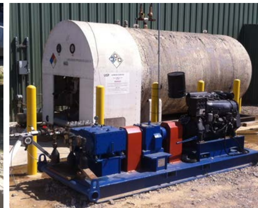
CO 2 Tank & HP Pump
