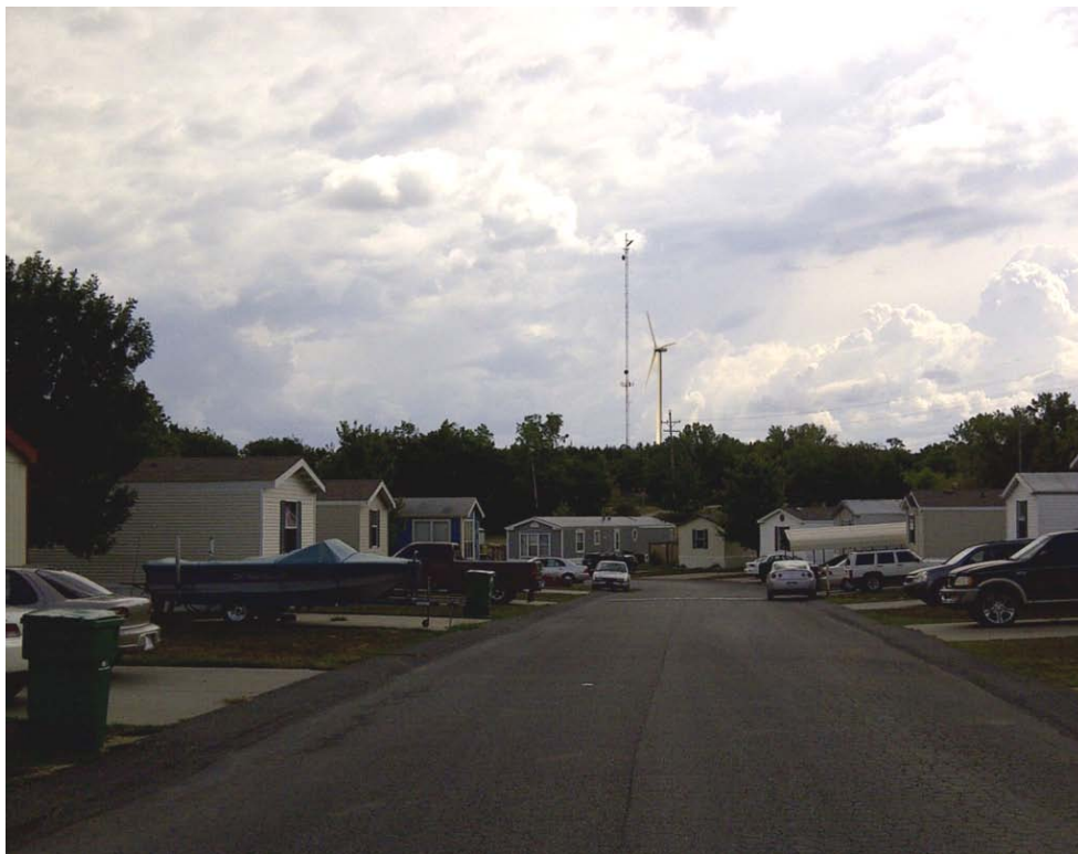
2: South view of turbine, communications tower, and power poles from River Chase Mobile Home Park.
