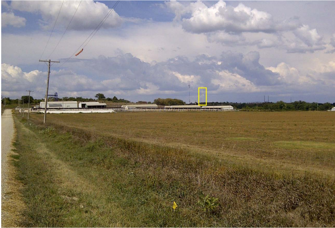
5: Northeast view of turbine and communications tower from College Avenue.
