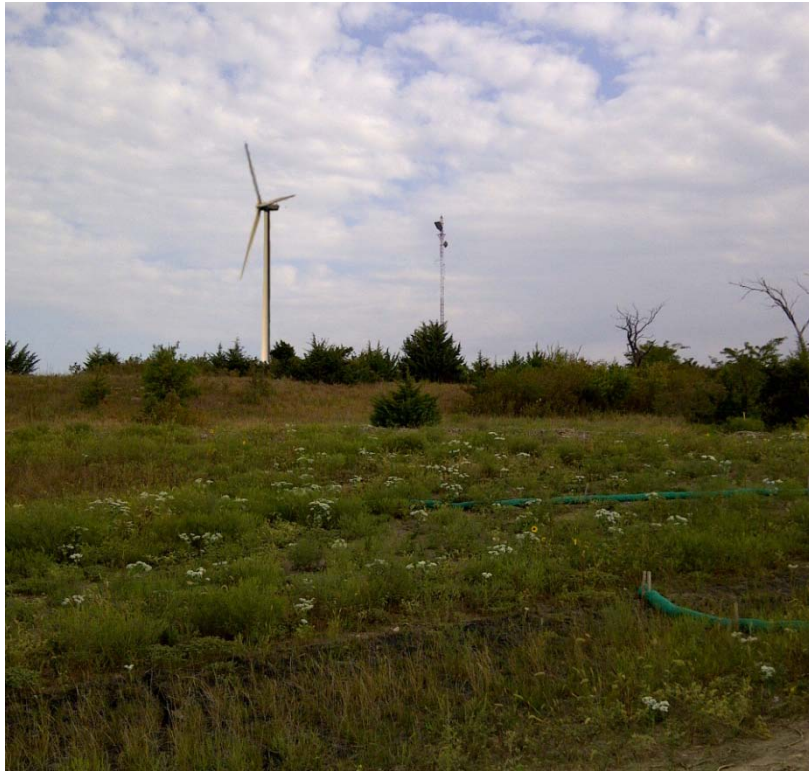
1: North view of turbine and communications tower from Westar Energy Substation.
