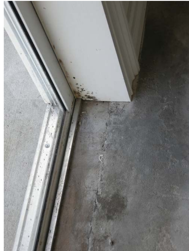
Mold on drywall at bottom of door
