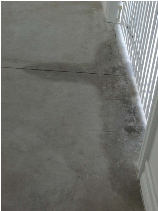
Water on floor from door condensation
