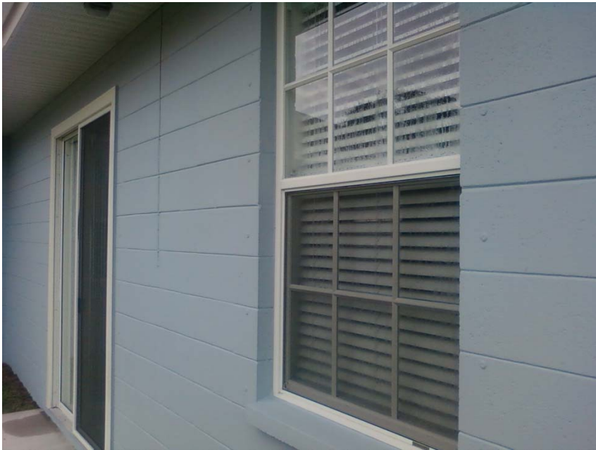
Condensation on all windows of tight building
