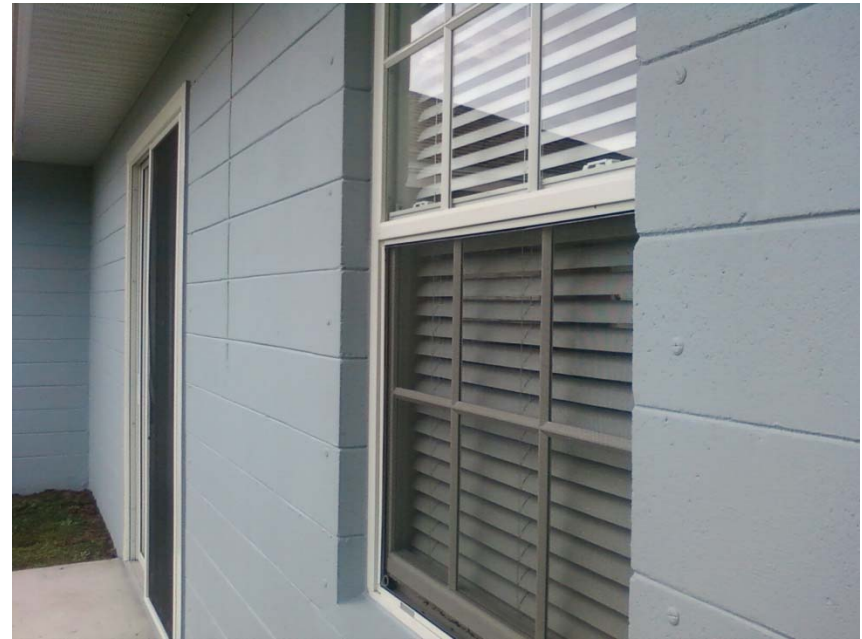
No condensation on windows of leaky building
