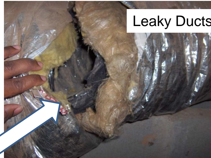
Significant attic infiltration
