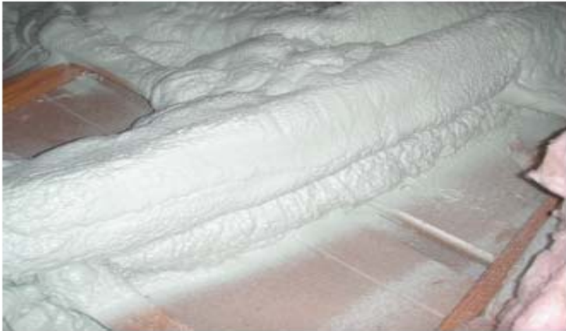
Figure 20. Ductwork well-sealed to sheetrock with ccSPF
