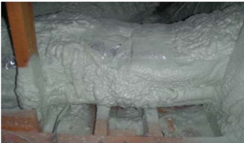
Figure 22. Varying thickness of ccSPF and interference from cross bracing
