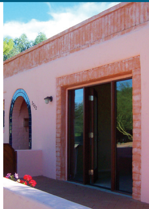
Miller placed rigid foam insulation and a new three-coat stucco finish over the original adobe walls but kept the historic masonry parapet visible to retain the home's southwestern character.
