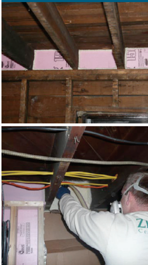
The Building America Asdal case study illustrated the use of rigid foam sealed in place with spray foam to insulate the band joists (top) and the use of spray foam around piping and wiring holes ( www.eere.energy.gov/buildings/building_america/cold_case_studies.html ).
