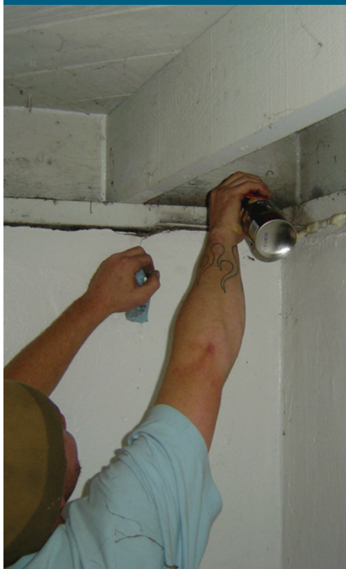
Sealing air leaks may result in a need for ventilation.
