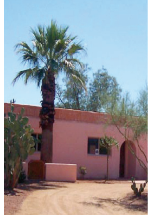
The Building America Tucson Adobe case study retained the historic landscaping with plants and ground cover that require minimum irrigation ( www.eere.energy.gov/buildings/building_america/hot_dry_mixed_case_studies.html ).
