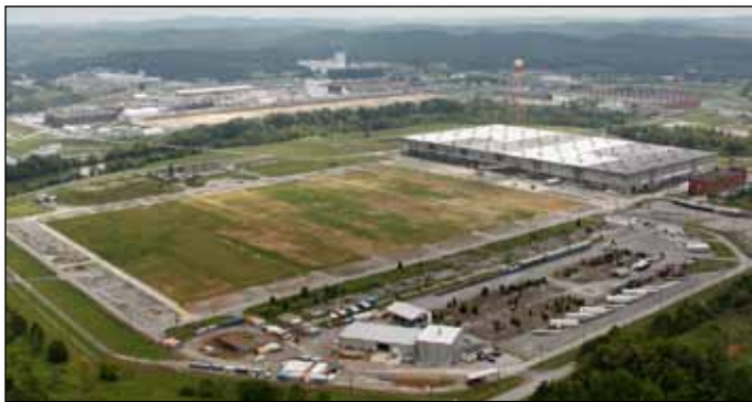
Aerial photo of Building K-33 site after demolition.
