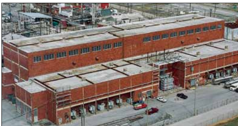
Using savings from other Recovery Act projects, the Beta-3 building at Y-12 will be characterized for contamination prior to eventual demolition.
