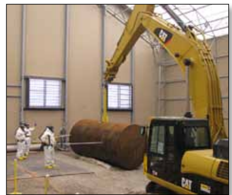
Workers practice tank removal inside the Tank W-1A enclosure.
