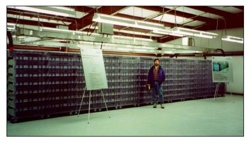
Figure 70. 1-MW/1.5-MWh Lead-acid Carbon System at Metlakatla, AK<sup>46</sup>
