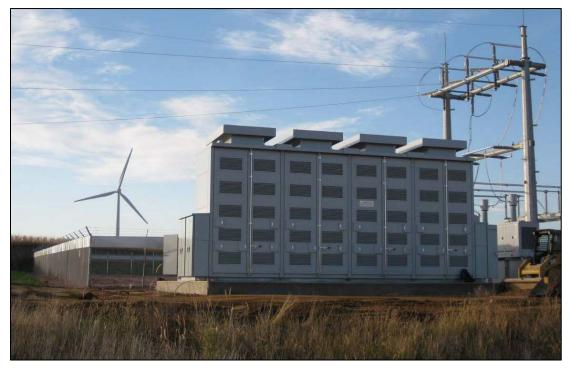
Figure 34. Xcel Battery Supplementing Wind Turbines, Lucerne, MN
