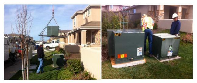
Figure 99. A 30-kW/34-kWh Distributed Energy Storage Unit (Being Installed and Inspected at the Sacramento Municipal Utility District's Anatolia SolarSmart Homes Development. Suppliers are SAFT, Grid Point, and Power Hub)
