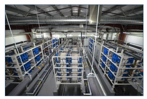
Figure 46. Prudent Energy 600-kW/3,600-kWh VRB-ESS Installed at Gills Onions, Oxnard, CA The system consists of 200-kW modules providing a total of 6 hours of electrochemical energy storage.
