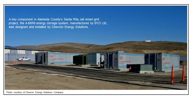
Figure 98. A 2-MW/4-MWh Li-ion Energy Storage System
