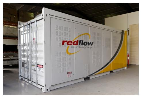
Figure 57. A 90-kW/180-kWh Zinc-bromine Energy Storage System by RedFlow (Housed in a 20-foot shipping container)
