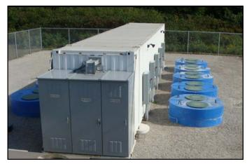
Figure 90. 1-MW Smart Energy Matrix Plant (Photo courtesy: Beacon Power)
