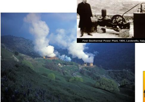
Dry steam plants use steam as the primary geothermal fluid. The steam is produced from the reservoir, which directly turns the turbine, that drives the generator to produce electricity. This geothermal technology is the oldest and dates to 1904, with the first documented generation of electricity in Lardello, Italy.
