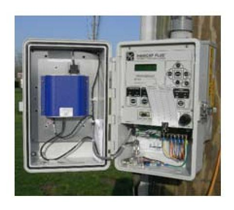
S&C Intellicap Control With SSN E-Bridge Radio for communications
