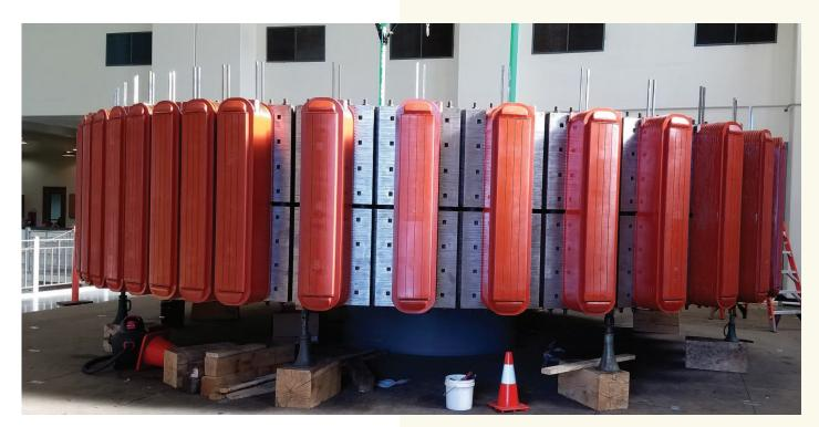
Refurbished poles and coils being installed on the rotating portion of Generator #2. Direct current flows in alternating directions to establish the machine's magnetic field.
