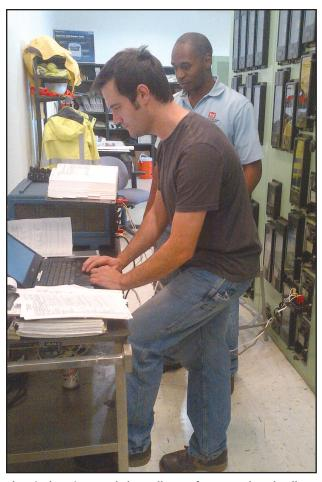
Electrical Engineers, Skylar Holloway, foreground, and Kellen Cole, verify and calibrate generator protective relay settings befind the Center Hill Powerplant control room switchboard.
