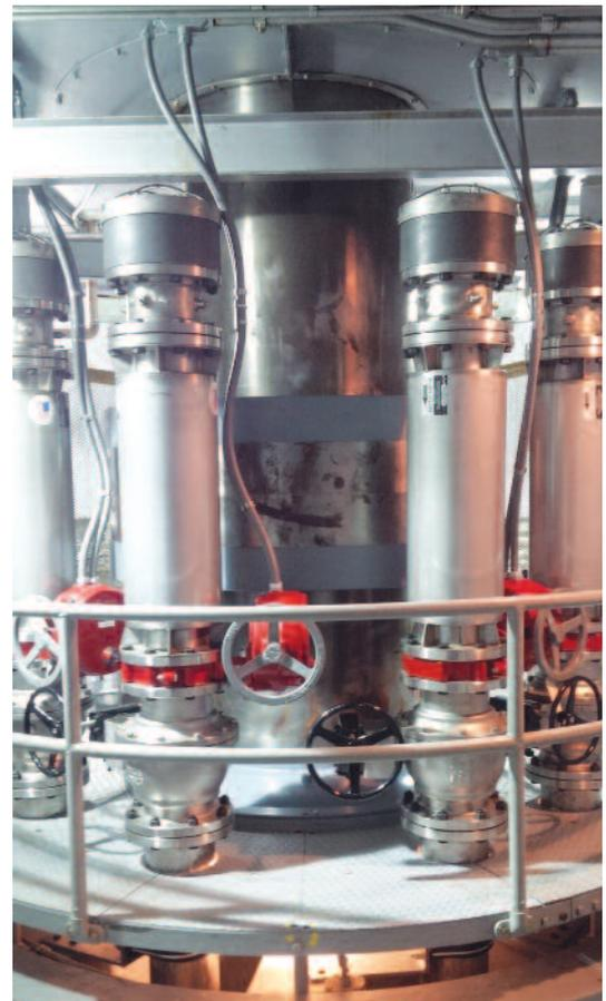
Brown Thornton representing Cumberland System Preference Customers in Kentucky and Mississippi poses in the Center Hill Generator 2 water passage next to new wicket gates and aerating turbine. As the turbine rotates, air is naturally drawn into hollow passages through valves and piping, shown in photo at right, to improve downstream dissolved oxygen levels.
