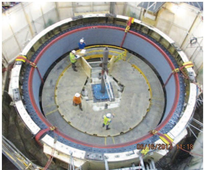
Carters Pump Generator 3 stator core replaced and ready to have new insulated conductors installed. The machine is scheduled to return to service in June 2018.
