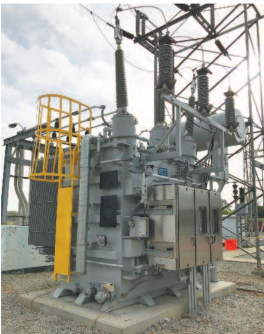
New main power transformer installed in the Miller's Ferry switchyard stepping-up voltage from generator to transmission system.
