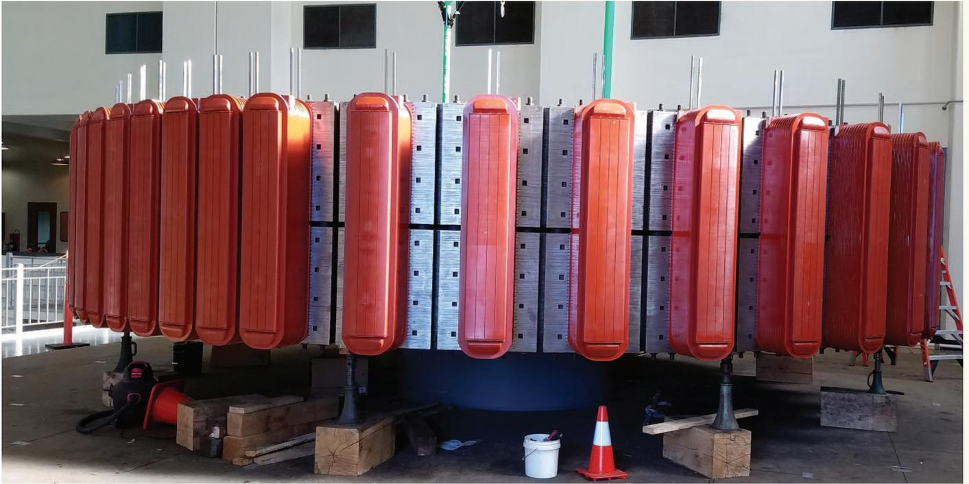
Refurbished poles and coils being installed on the rotating portion of Generator #2. Direct current flows in alternating directions to establish the machine's magnetic field.
