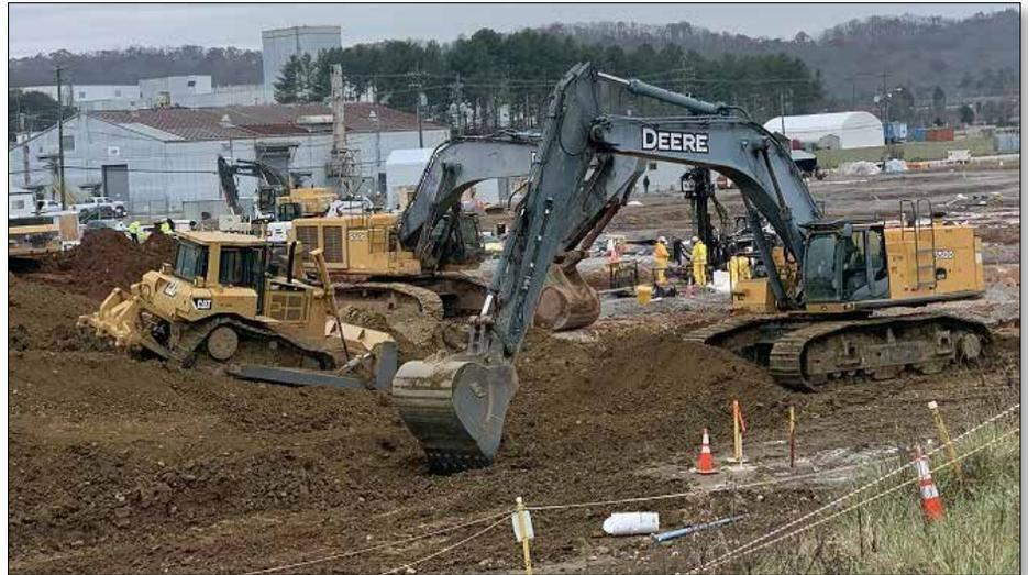
*Workers have completed an excavation of contaminated soil from the K-25 footprint, removing more than 90,000 cubic yards of soil.*
