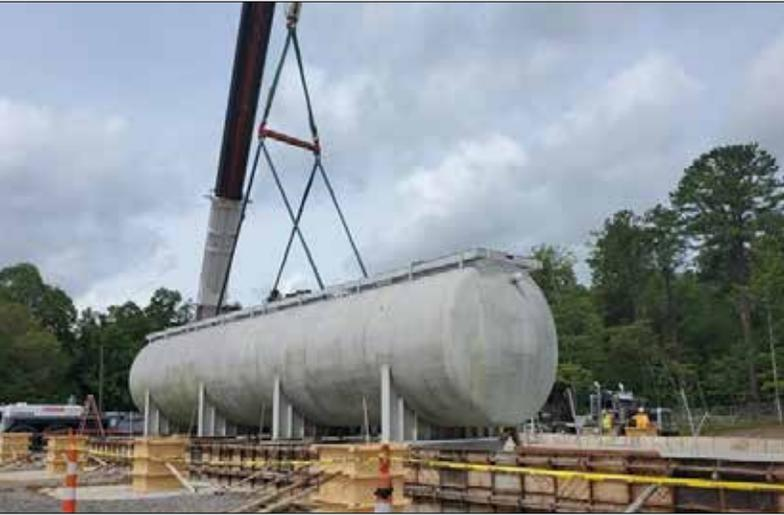
*Crews moved a massive 50,000-gallon tank into position to support efforts at the Sludge Processing Mock Test Facility under construction at Oak Ridge.*
