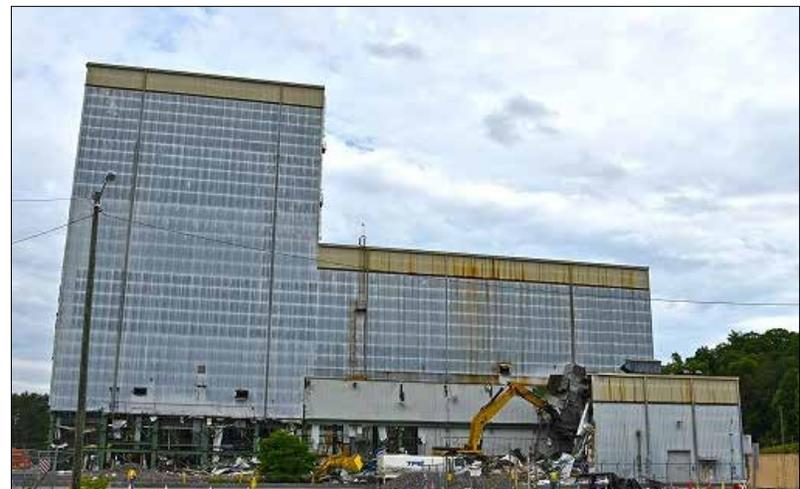
*At 180 feet tall, K-1220 was too tall to be safely torn down with conventional heavy equipment, so it was torn down using giant winches.*
