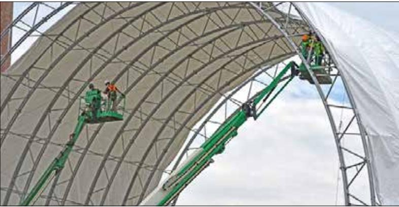
*Crews are manually adding 12,000 square feet of fabric to the trusses to complete the cover for the protective tent at the Building 3026 demolition project at Oak Ridge.*
