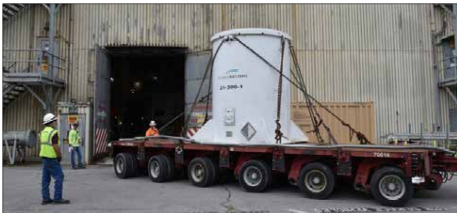
The reactor vessel of the Oak Ridge Research Reactor is loaded into a protective shipping container for transportation and disposal offsite.
