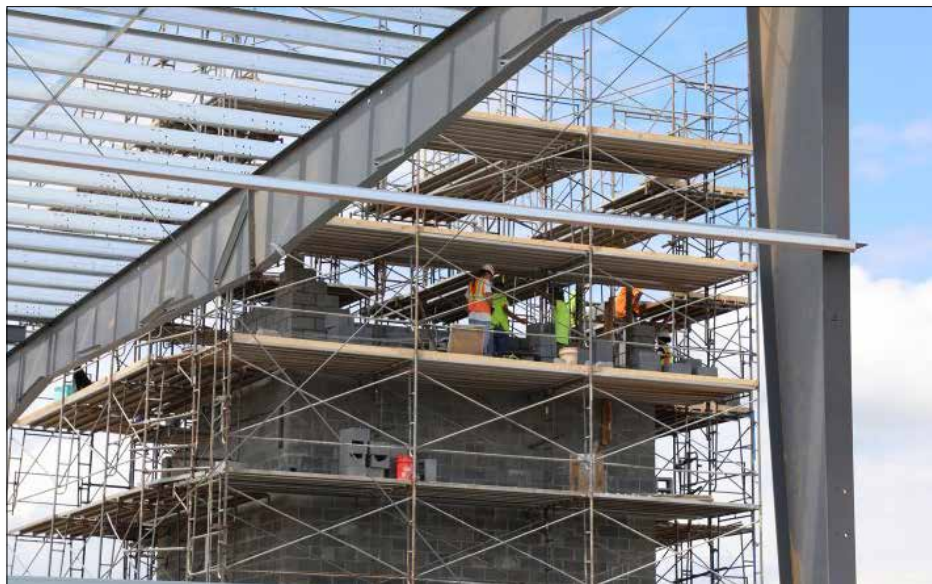
The K-25 Viewing Platform is taking shape with construction crews from Geiger Brothers finishing the concrete slab and erecting the structural steel framework. Construction is expected to be complete next spring.
