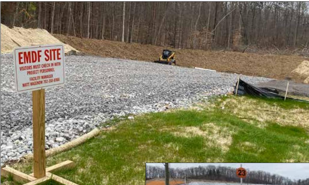
*Left: Early site preparation for EMDF is expected to be complete this spring. The second construction phase will include a groundwater field demonstration study located on a portion of the final footprint of the site. Oak Ridge will gather data for two wet seasons to inform final design choices for the facility.*
