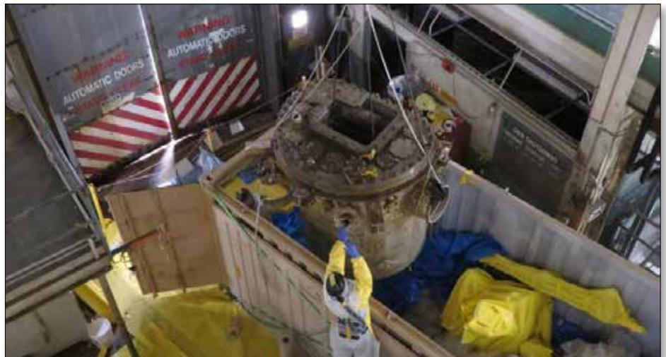
*Workers in the Oak Ridge Research Reactor facility remove the top portion of the reactor vessel for disposal. They will remove the next portion of the reactor vessel this year.*
