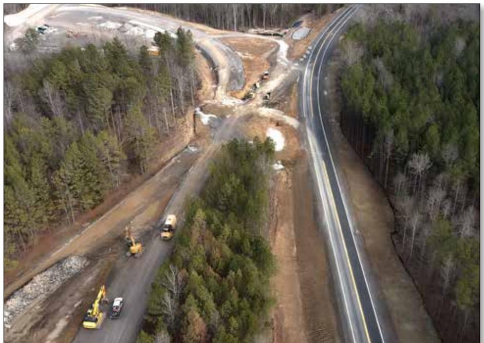
*One of the major tasks involved with site preparation and construction of EMDF involves moving Bear Creek Road and Haul Road to accommodate the site design.*
