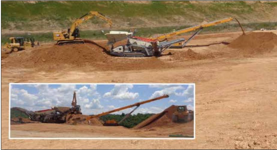
*Large machinery, known as a soil screener, removes rocks to ensure the construction of the Landfill V expansion meets clay liner requirements. The Landfill V expansion project is on schedule to be completed by the end of the year.*
