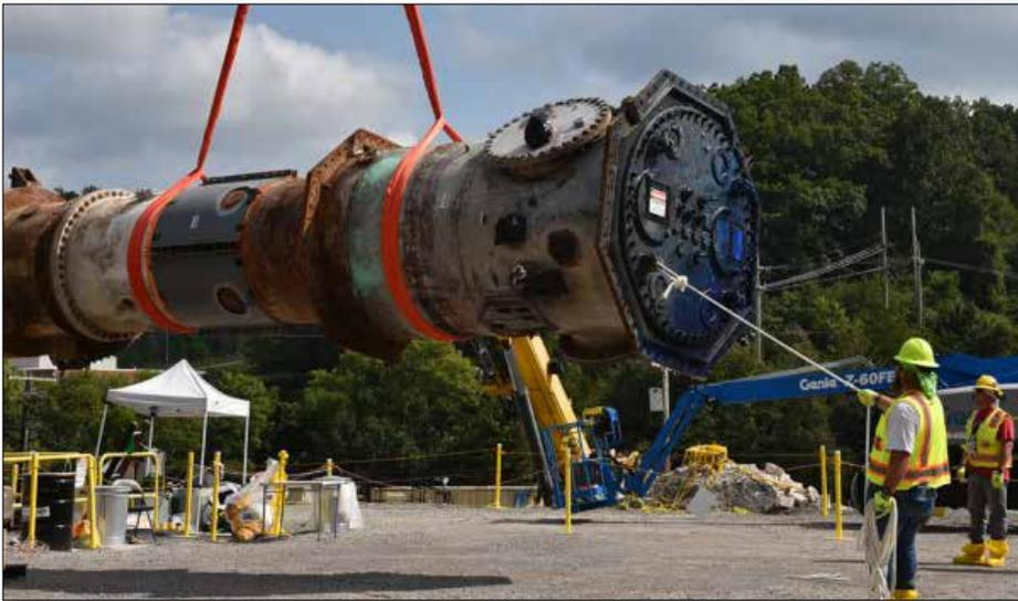
*In the final step of the Low Intensity Test Reactor demolition project, a crane raised the 37,600-pound reactor structure from its housing, placing the 30-foot-long reactor vessel in a specialized carbon metal container for shipment for disposal.*
