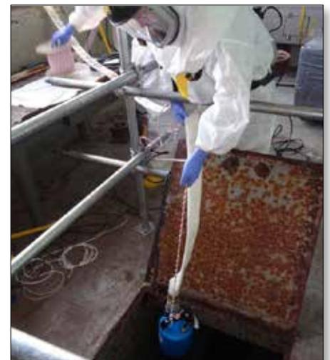
*A worker lowers a hose to pump water from the basement area of the Beta-1 facility. Crews pumped 1 million gallons over the 42 work days.*
