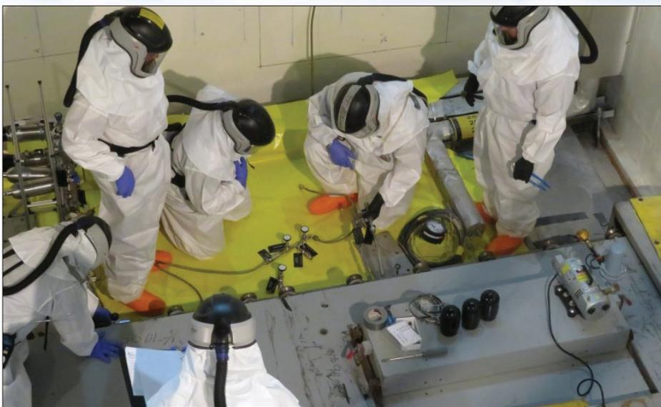
*For the first time in 26 years, EM crews performed sampling of gases produced as byproducts at the Molten Salt Reactor Experiment at Oak Ridge National Laboratory. This work could not occur until new piping and safety features were installed at the facility. They have performed five samples since December.*
