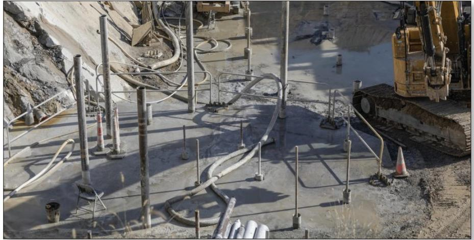
*ORSSAB members recommended fully funding work on the Mercury Treatment Facility as part of the board's broader recommendation for OREM's FY 2025 Budget Priorities. Above, Oak Ridge construction crews installed micropiles to help lay the foundation for the headworks facility site for the Mercury Treatment Facility. They installed 79 micropiles, some going nearly 70 feet down, to provide structural foundation support for the headworks facility.*
