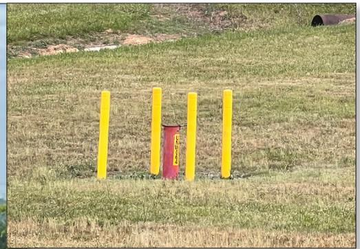
OREM uses monitoring wells like this one at ETTP to identify and track groundwater contents and quality.
