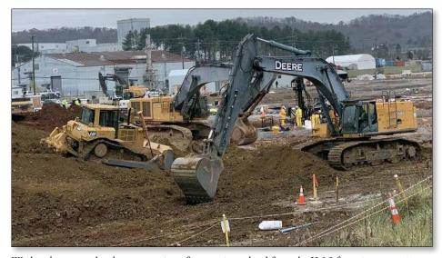
Workers have completed an excavation of contaminated soil from the K-25 footprint, removing more than 90,000 cubic yards of soil.
