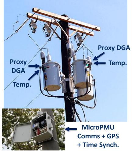
**New Low-Cost Sensors Integrated with MicroPMUs**
