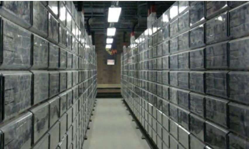
LEAD-CARBON BATTERY STACKS AT EAST PENN MANUFACTURING PLANT
