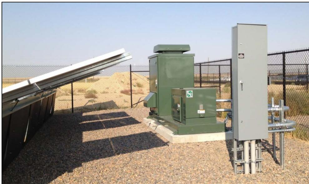
**Figure 40. Containerized 25 kW/50 kWh FIAMM Battery Unit (large green housing) on Concrete Pad, Next to S&C PureWave CES (small green housing)**
