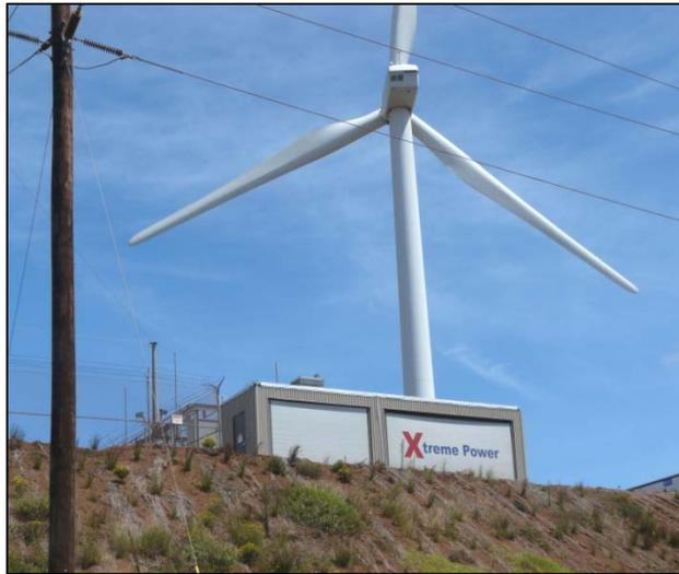
**Figure 72. 1.5-MW/1-MWh Advanced Lead-acid Dry Cell Systems by Xtreme Power in a Maui Wind Farm**
