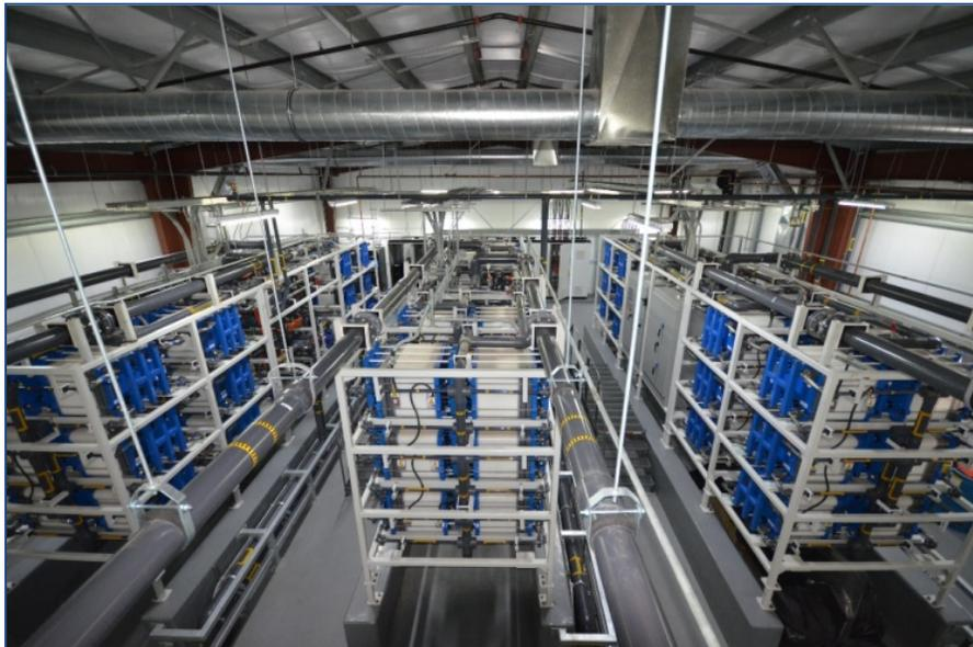
**Figure 46. Prudent Energy 600-kW/3,600-kWh VRB-ESS
