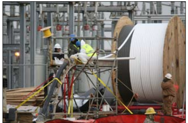
Triax cable being pulled into the underground duct at Bixby substation.
