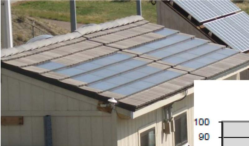
Ventilated counter-batten installation produced 3.4% more direct current (DC) power than the direct-mount installation
