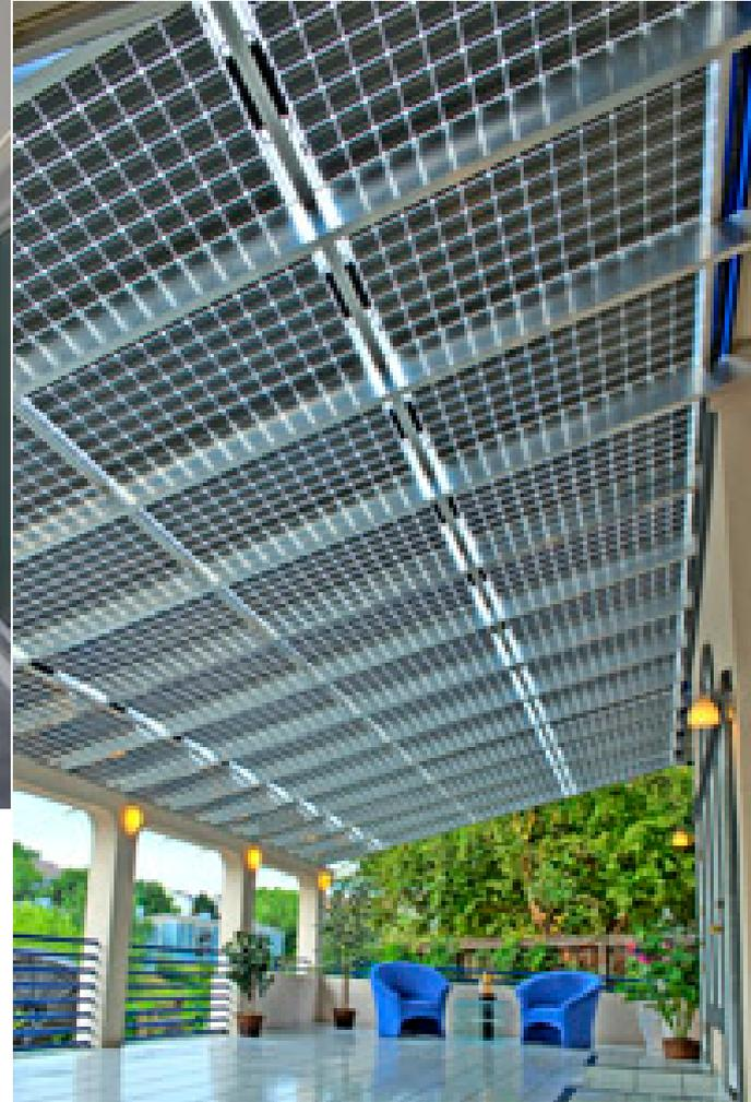
All of the 962-ft<sup>2</sup> porch roof is comprised of 69 solar panels that don't sit on top of the roof; they are the roof. The completely watertight structure allows about 15% of natural light to filter through the panels, lighting the space below. All wiring is hidden within the canopy's aluminum support beams.
