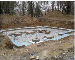
Four inches of rigid foam will wrap the slab perimeter while an additional 8 inches (R-35.6) of high-density EPS rigid foam will extend under the entire slab.
