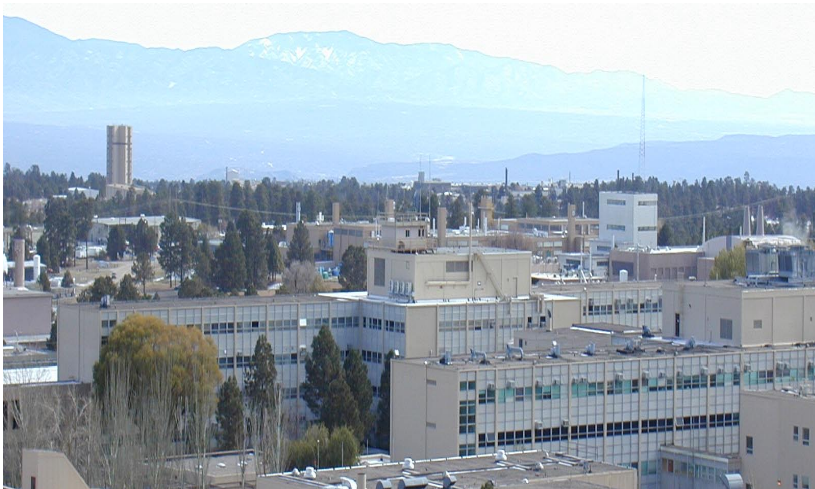
Figure 3a. Existing Administration Building 3-43 (looking mostly east).
