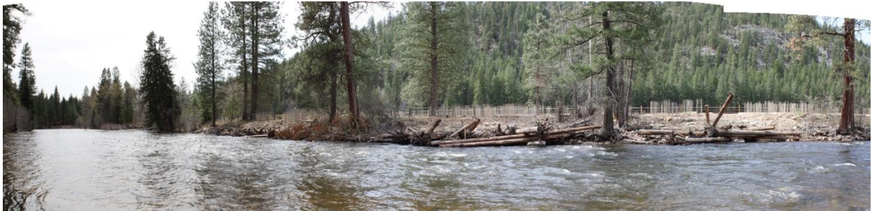
Figure 39: Photograph of constructed log structures on the south end of Eightmile Ranch riverfront. The vertical members on the right-hand side of the photo meet scenic quality objectives because of there are only two, and they have different heights and angles.
