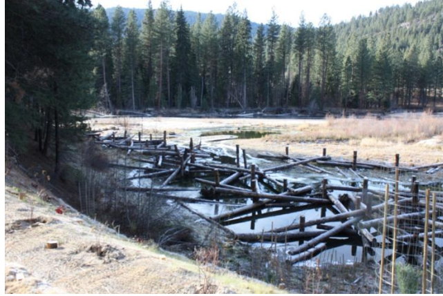
Figure 42: View of Structure 13B from the East Chewuch Road.
