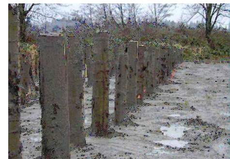
Example - Live Cottonwood Flood Fence (after first flood) - B. Aldrich, Snohomish County, WA
