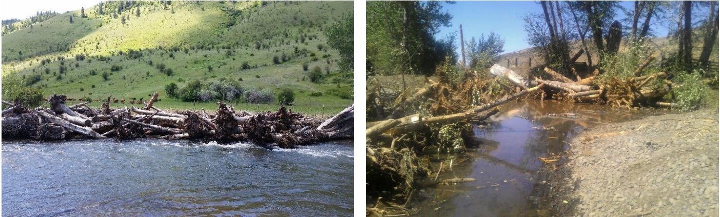
Figure 2. Examples of what large wood structures may look like once installed along this reach of the GRR.
