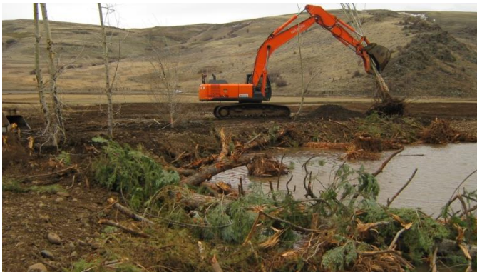
Figure 3 – 300 series Track-mounted excavator
