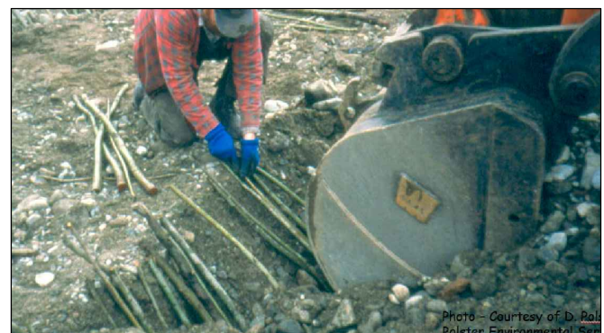
Willow Trench Construction
