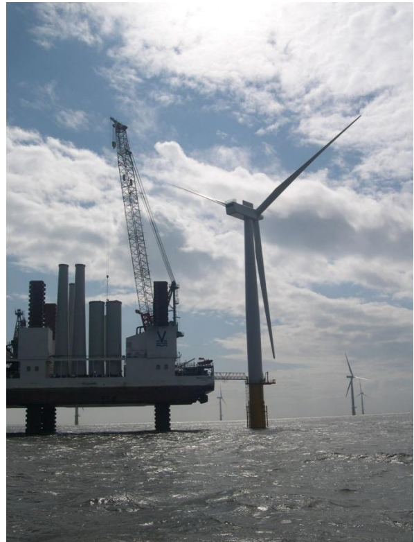
Figure 3-1: WTG typical installation.
