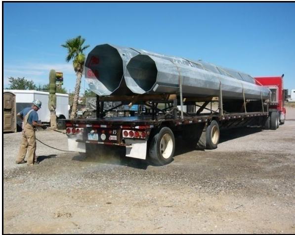
Photograph 2-7 Example of Truck Delivery to Assembly Area
