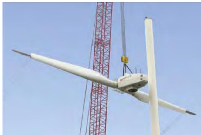
Installing nacelle and blades in one pick.
