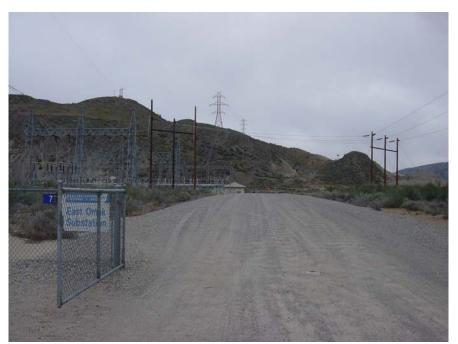
Photo 1. View from the Cobble Road entrance to the East Omak Substation, facing north; the area where fiber would be installed is the strip of vegetation on the right side of the photo, conduit would be installed under the gravel entry road into the small building (BPA control house) in the distance.
