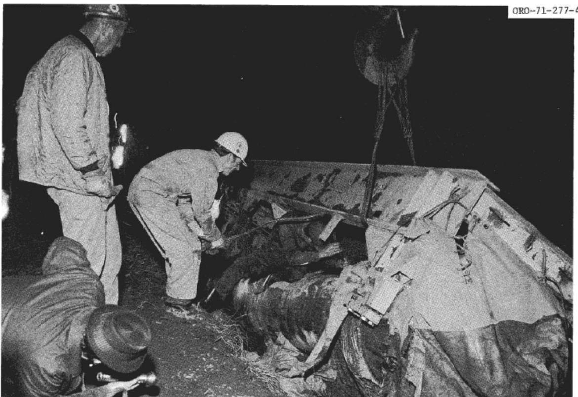
**Fig. 4-4. Initial lift during cask retrieval (Chandler 1972).**
