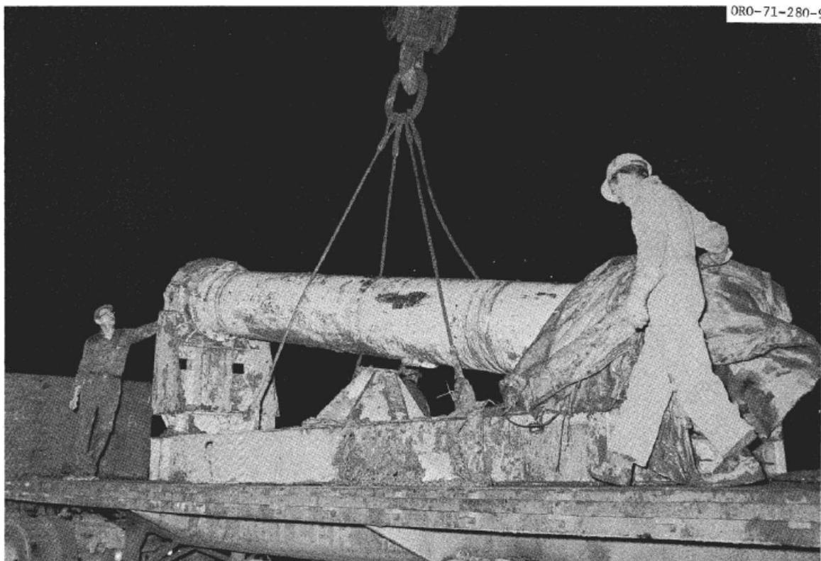
**Fig. 4-5. Cask placed on trailer (Chandler 1972).**
