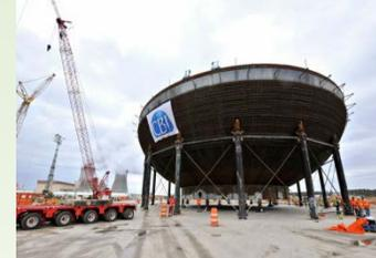
*Vogtle Unit 3 Nuclear Island showing nuclear island basemat pour and Containment Vessel with exterior rebar installed (Courtesy of Southern Company)*
