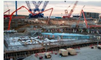
*VC Summer Unit 2 Lower Bowl Assembly and nuclear island concrete placement (Courtesy of SCANA)*
