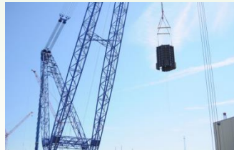
Placement of unit 3 CA04 module; arrival of unit 3 reactor vessel (Courtesy of SCANA)
