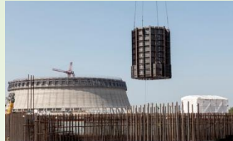
Placement of Unit 4 reactor cavity module; progress on unit 3 and 4 cooling towers (Courtesy of Georgia Power/Southern Company)
