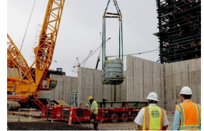
Vogtle 4 step-up transformer is lifted into place. (Courtesy of Georgia Power/ Southern Company, May 2018)
