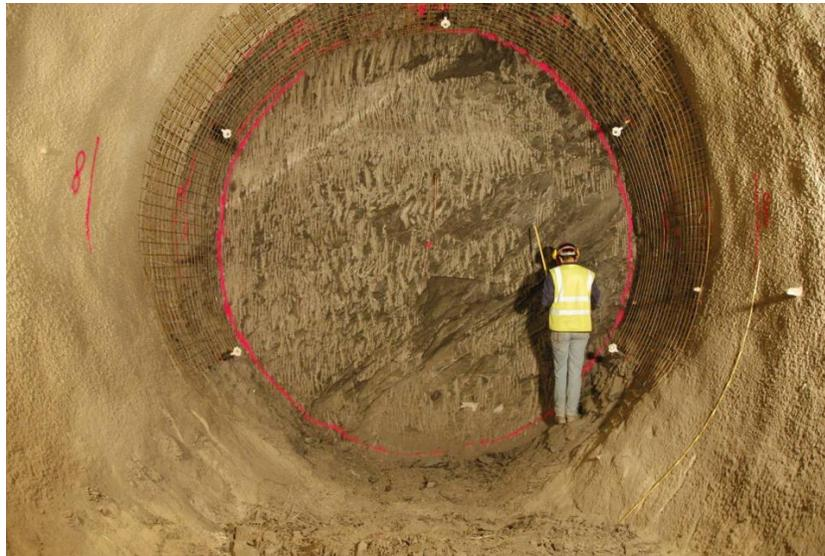
**Figure 3-5.** View of FE tunnel face from the FE niche showing beddings dipping  $45^\circ$  (Vieter, 2012).
