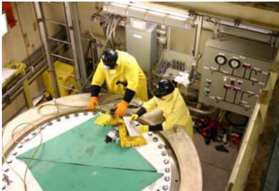
Figure 3-3: Lid Installation of a TN-32 Cask.
