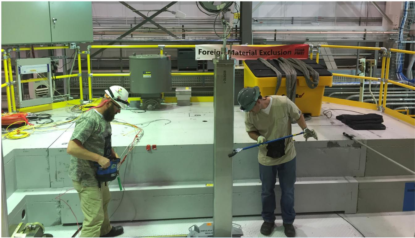
**Figure 2.** Insertion of an experiment vehicle containing three gadolinium-SPNDs into the TREAT reactor.
